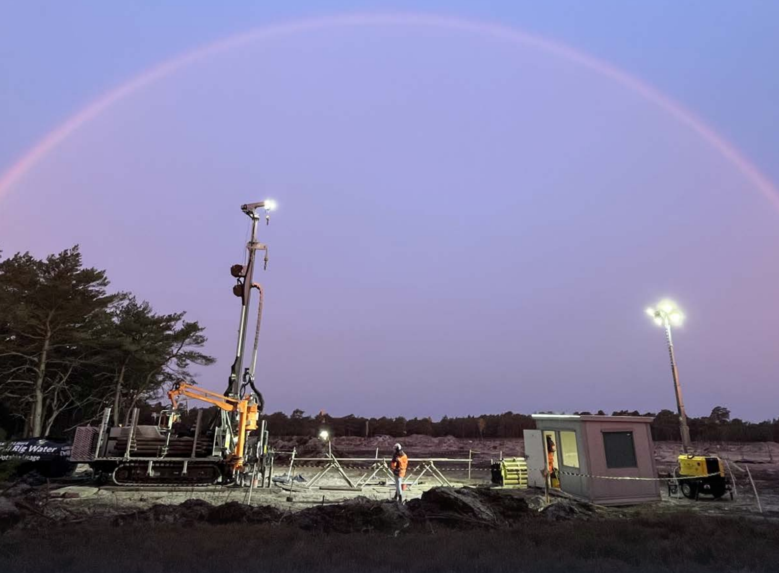
Drilling with the LRS 275 in Poland
