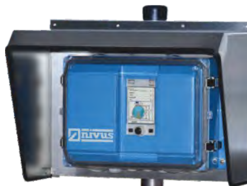
Field enclosure installation
