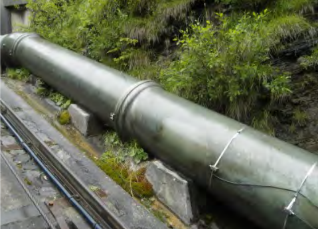
Turbine intake flow measurement using clamp-on sensors
